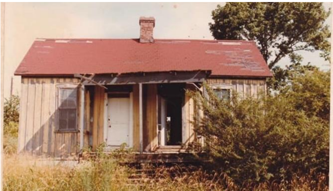
Laborer Section Houses
