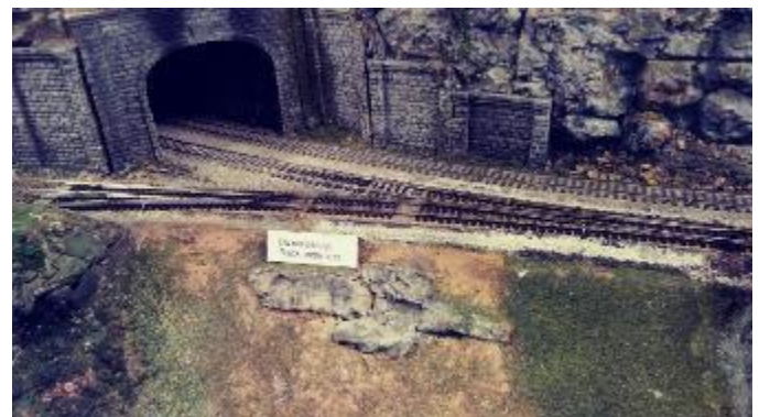
New track installed at the south end of the Ramey tunnel
