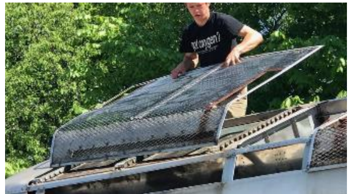
A HOBO Railroad volunteer secures a grate over the fan housing
