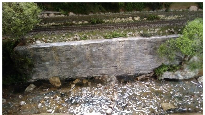
Looking at the retaining wall in the upper reaches of the Doe River gorge... prior to pouring the "water" he painted the river bottom, added pebbles and casting to represent rocks, and debris representing dead fall from the forest above the river.
