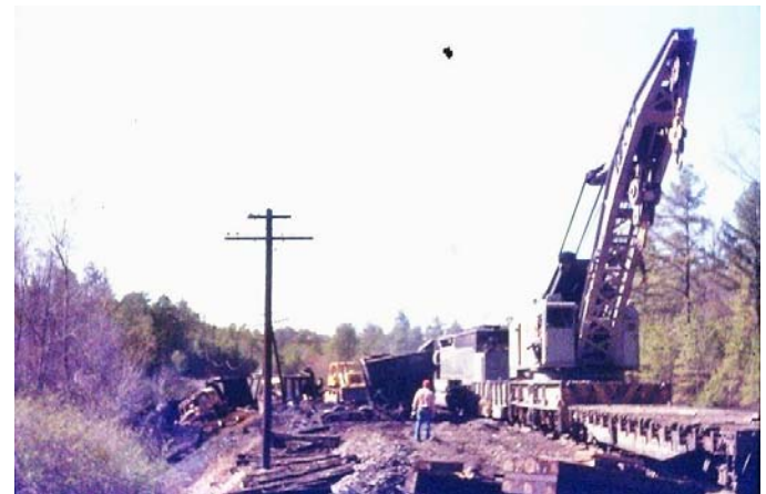
The efforts included calling out the big hook as well as the smaller MOW tractors... the second track to the left in the photo appears to require a total reconstruction of the right-of-way.
