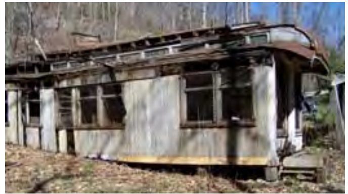
West Virginia Midland "Holly," a private office car, build in 1902 by Jackson & Sharpe, served the WV Midland and the Pardee Curtin Lumber Company in the mountains of West Virginia. This car is the only known narrow gauge office car with a southeastern heritage still in existence.
