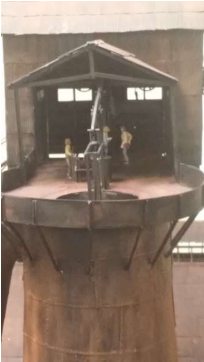
Blast Furnace Retort where a mix of Ore, Coke, and Limestone are loaded for heating
