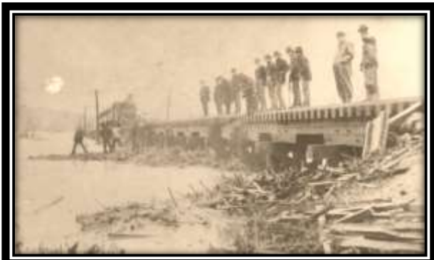
High water along the line in December 1926
