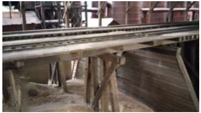
Interior of Materials Bays
