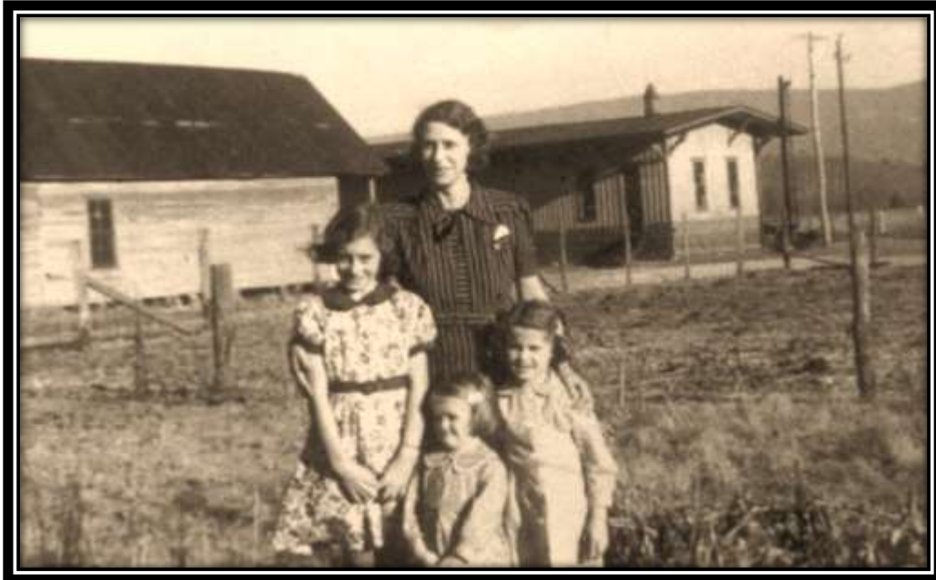
A Daus, Tennessee family is pictured here in about 1946. The old Daus passenger & freight depot can be seen in the background. This depot was later replaced with a waiting shed pictured below.
