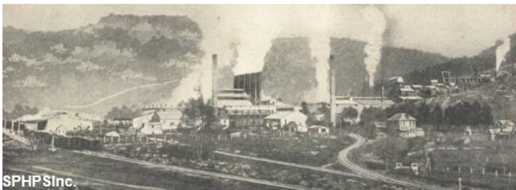
Penn-Dixie Cement Plant Switch Track Richard City, Tennessee Circa 1925
