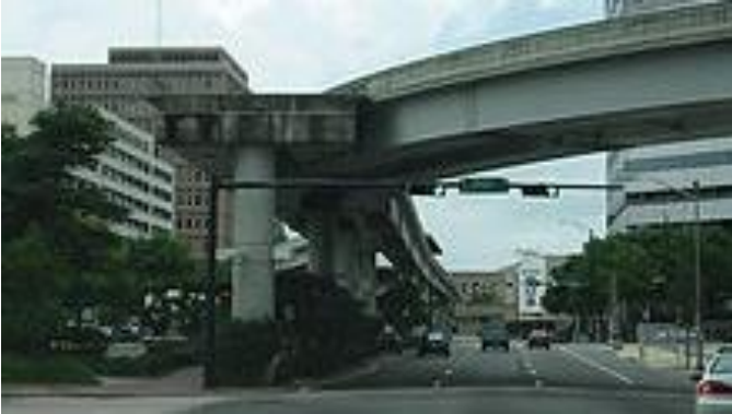
Skyway track curve between Central and Hemming Park stations at Hogan Street
