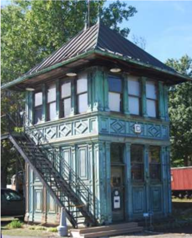
A vintage MTA control tower greets visitors as they pull into the museum's parking lot
