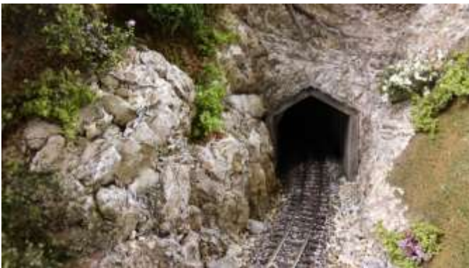
Fred Alsop completed building the tunnel portal and lining for tunnel 4 on the ET&WNC layout.
