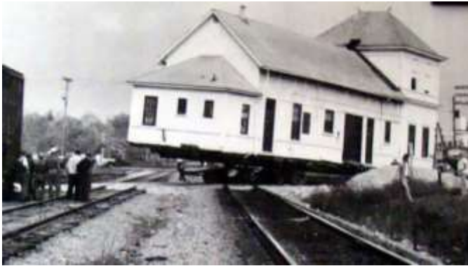
The depot once sat on the other side of the tracks but was moved to its present site in its entirety as seen in the photo above.
