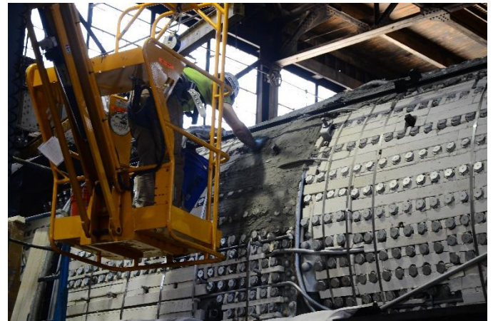
Replacing the lagging on UP 844
