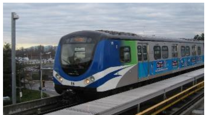
EXCEPT FOR ROUTES IN THE DOWNTOWN HUB, THE SKYTRAIN CRISS-CROSSES THE CITY ON ELEVATED TRACK AND DEDICATED RIGHT-OF-WAY.
