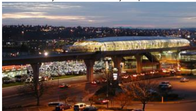
SKYTRAIN TERMINAL AT THE VANCOUVER AIRPORT
