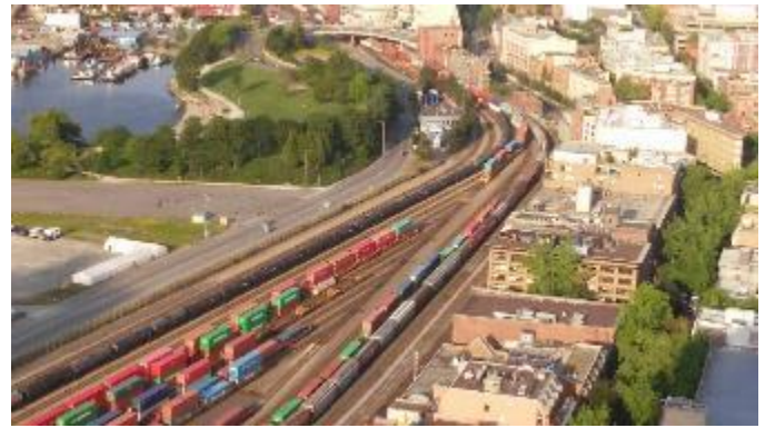
VIEW OF THE CP HARBOUR YARD FROM THE HARBOUR TOWER
