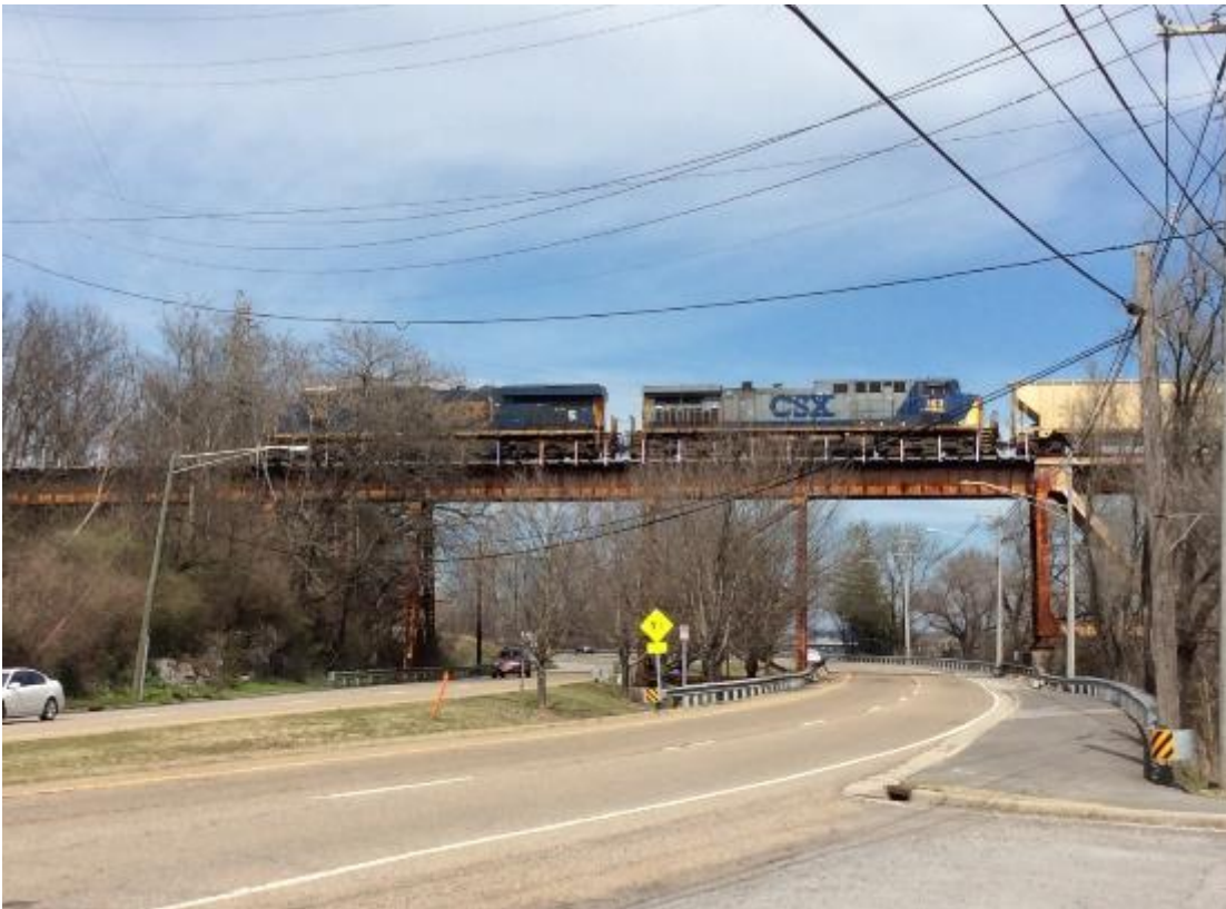
CSX mixed freight crossing the Tennessee River near the University of Tennessee's campus.
