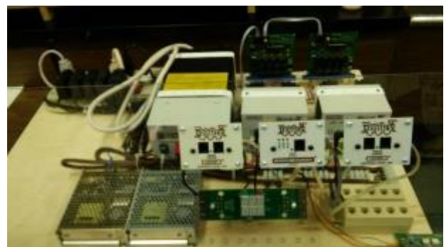
Frank Fezzie has been busy building the new electrical control center for the Tweetsie layout
