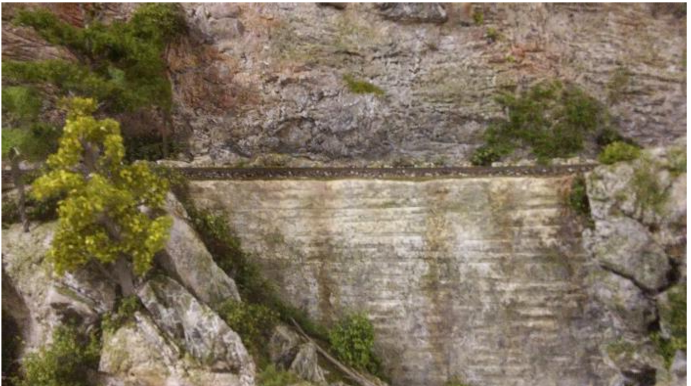
RETAINING WALL NEAR PARDEE POINT IN THE DOE RIVER GORGE
