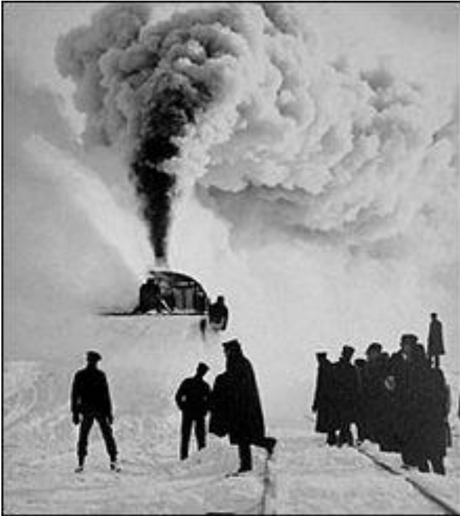
' A rotary snowplow at work in New Ulm, Minnesota.
