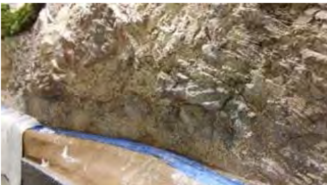
Some of the rock wall lining the Doe River Gorge
