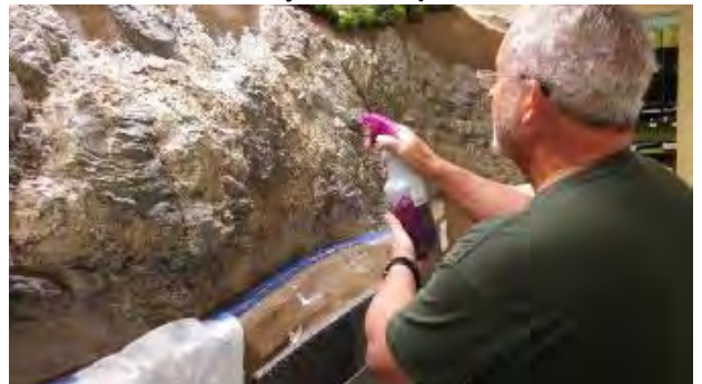
Fred is over-spraying the rock casting with a dilute black spray to bring out the highlights of the carved rock facing
