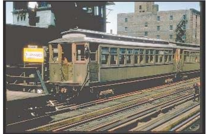
A lot of ex-Met wood cars finished out their service by wood cars on the Ravenswood, the Stock Yards and the Kenwood lines. On the last days of the Kenwood, all of cars were numerically above 2900. Car 2904 is seen working the Kenwood branch, stopped at Indiana in 1957. The line (and cars) was taken out of service by the end of the year; 2904 was scrapped in May 1958.
