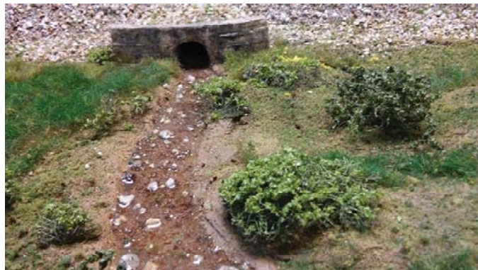
Culvert under the big fill south of Shell Creek
