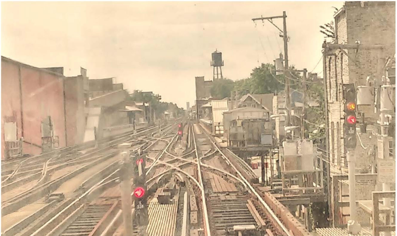
These two views are from the front of car 3283 heading towards the Loop. Notice the complex track work with three sets of double crossovers and the requisite diamonds. This complex track arrangement is required to accommodate trains running on multiple routes against local and express traffic.
