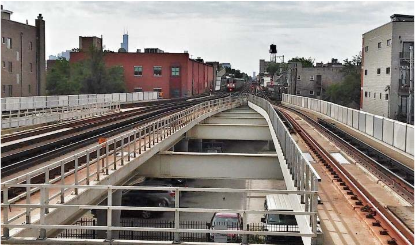
Here is a view of the "L" structure from the top side. The view is looking south toward the Loop from the end of the Belmont platform. Note how even the lower level of the right-of-way is used as a car park. Parking in the city runs upwards of $30 per day especially in the Loop itself.
