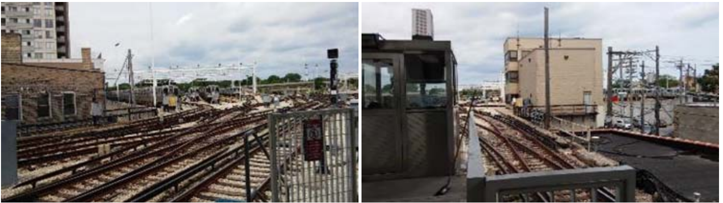
A view of the Howard Street yard, home for Skokie, Evanston and Loop trains.
