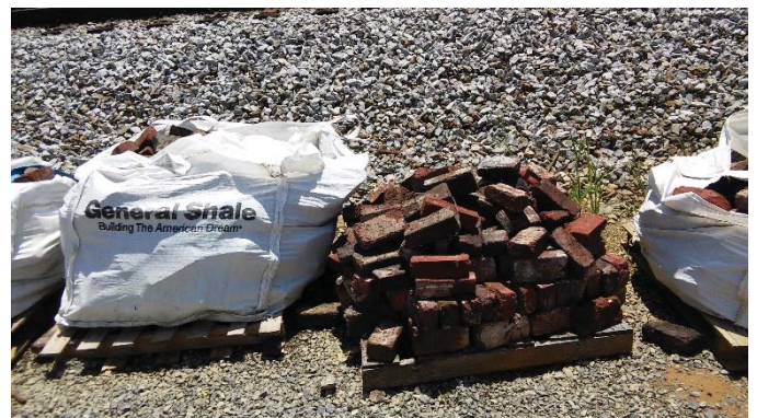
Paving bricks have been saved for reconstruction of the station platform.
