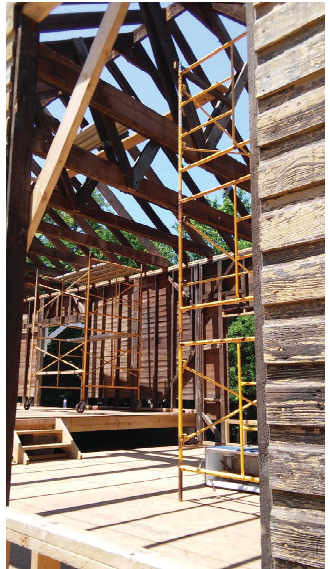
A view of the interior reveals the freight/baggage section sat on a raised platform above the passenger/office section of the station.
