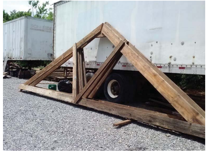
Roof trusses reassembled ready for setting in place
