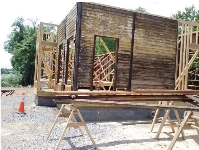
East end of the station being reassembled
