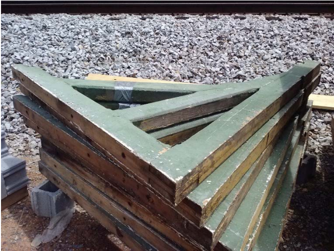
Braces for the overhanging eaves appear in good shape
