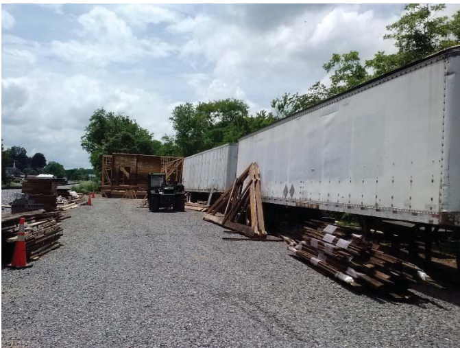
Two of the three trailers used to store pieces of the station
