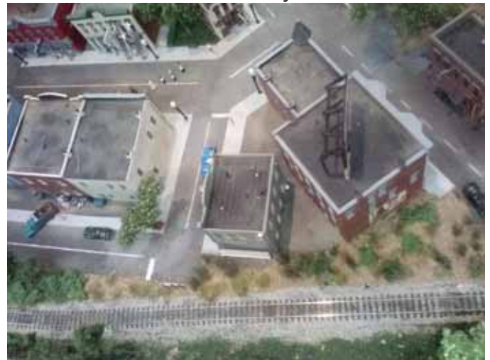
A rooftop view of the downtown business district
