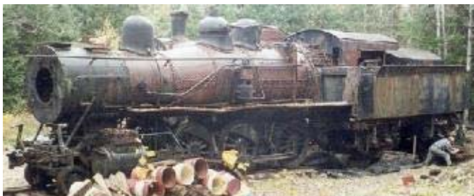
Volunteer members of the Allagash Alliance transported hand jacks and dozens of buckets of ballast (heavy gravel) to the remote site then leveled the tilting locomotives by hand.
