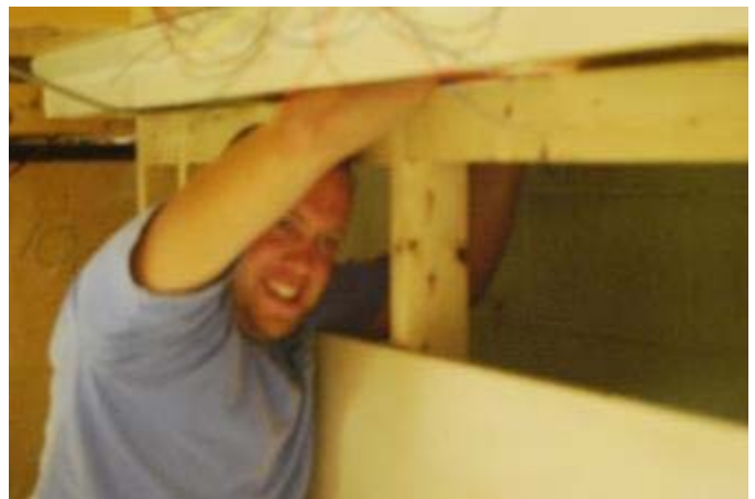
Jesse plays at being a contortionist underneath installing Tortise switch machines in the Johnson City yard portion of the layout.
