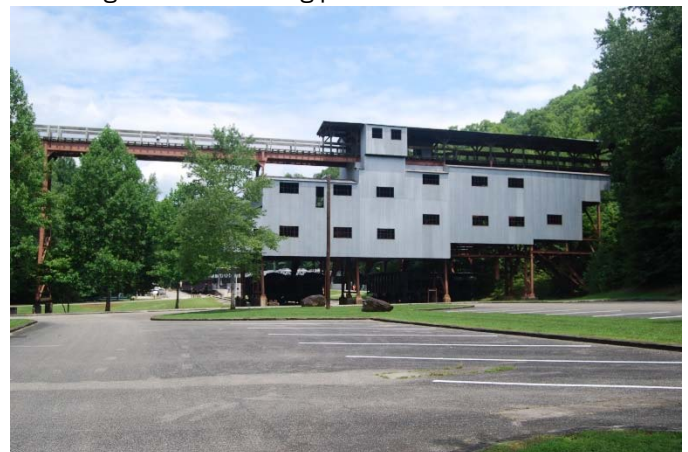
From the Mine the coal was transported to the crusher pictured above. There the chunks of coal was washed, broken into smaller pieces, screened for size and sorted to storage bins. From there the coal would be loaded into the awaiting railroad hoppers for transit to the coals final destination.
