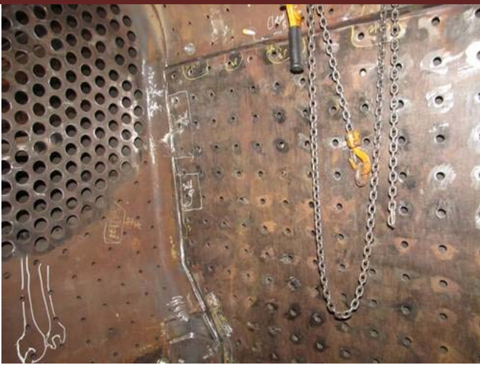
Front flue sheet cleaned and ready for flues - July 10, 2012
