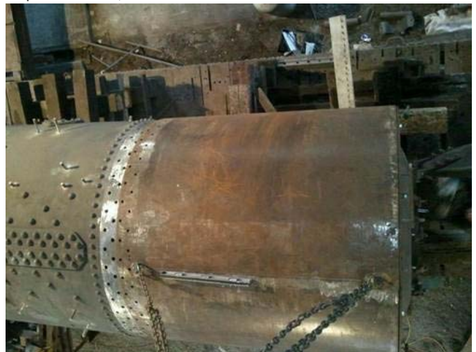
Fitting smoke box to boiler - January 29, 2013
