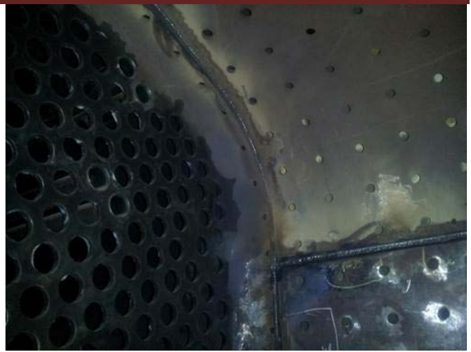
Lower front flue sheet patch has been welded in place - August 9, 2012
