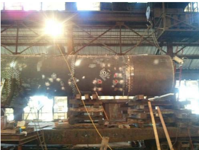
Leo and Tom of Wasatch Railroad Contractors threading stay-bolt holes.
