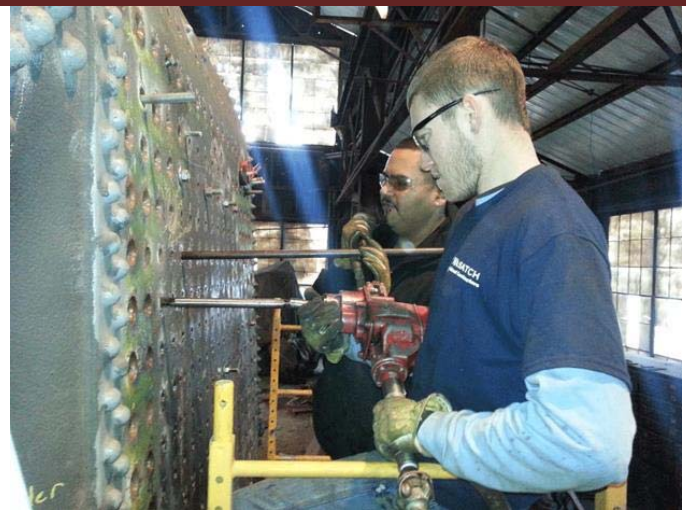
Installing front tube sheet rivets is a group effort!
