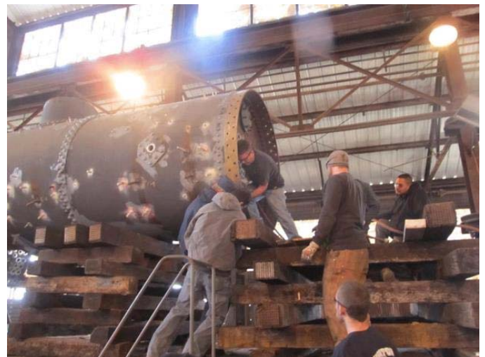
More and more tubes in the boiler!
