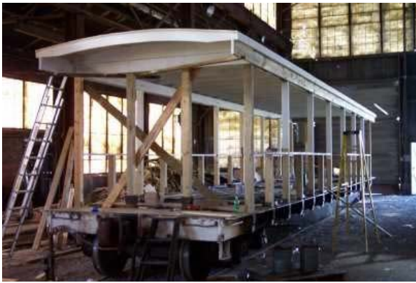
Car #1003 framed and under roof on September 18, 2003
