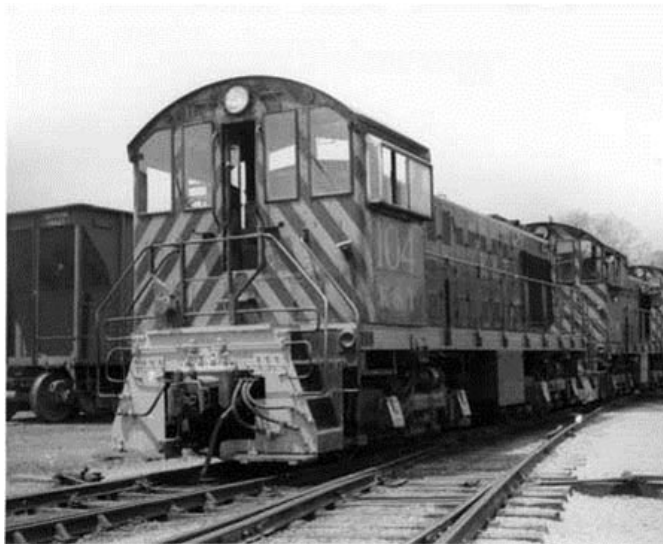
Kentucky & Tennessee Railway #104 1944, BB, built by ALCo, 1000 hp. Ex-D & H 3028.
