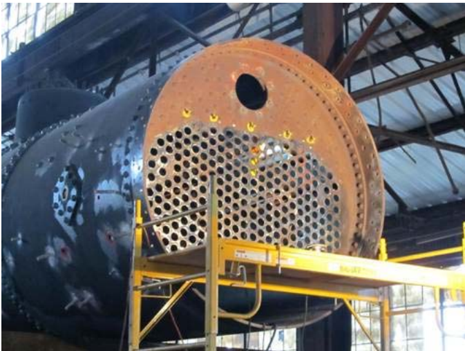
K&T Superintendent Don Powell checks on the work being performed July 10, 2012
