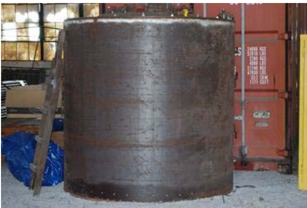
Hanging new firebox side sheets, May 11, 2012
