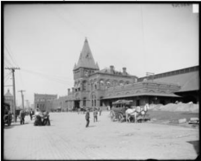
View of the Second NYC Depot in Rochester
