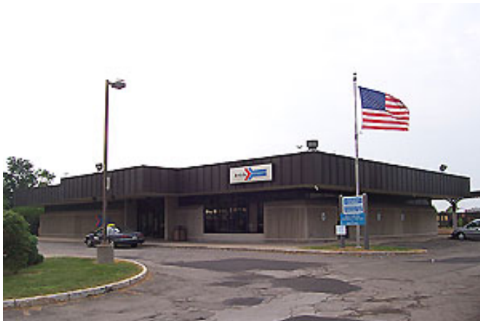
The Station Building as viewed from the street entrance.
