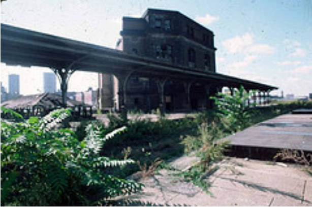
Demolition of the Bragdon Station
