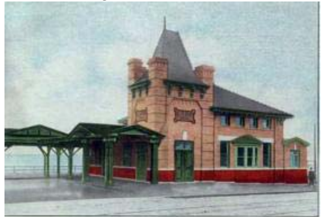
Looking South from Court Street.
