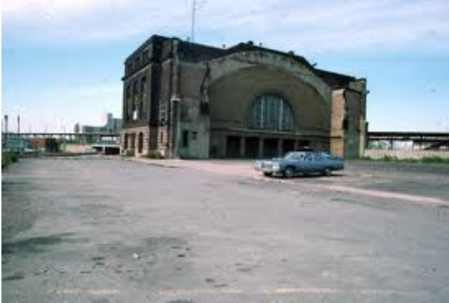
Demolition of the Bragdon Station
