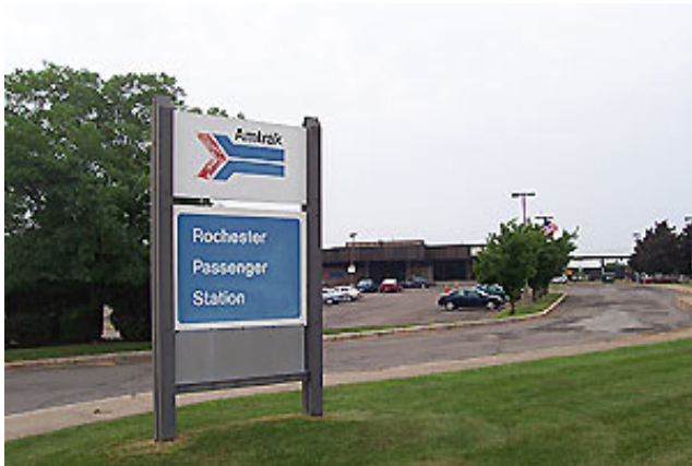
Entrance to the Station Building in 2005
