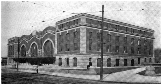
Exterior View of the New York Central Station at Rochester
