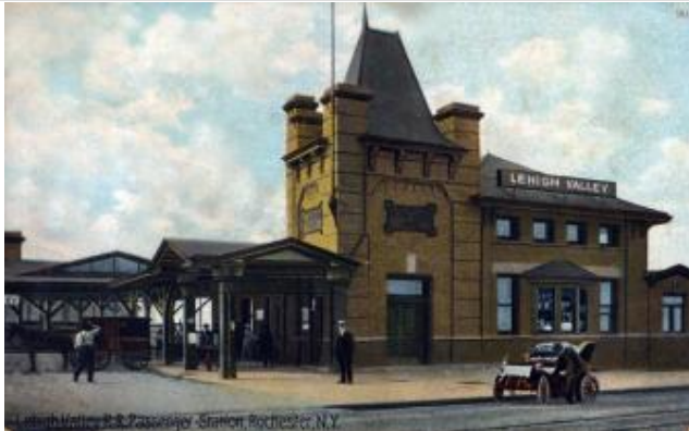
Looking South from Court Street.
