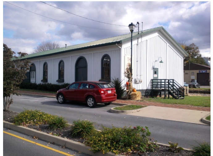
Freight House - 3/4 View Northwest Corner
