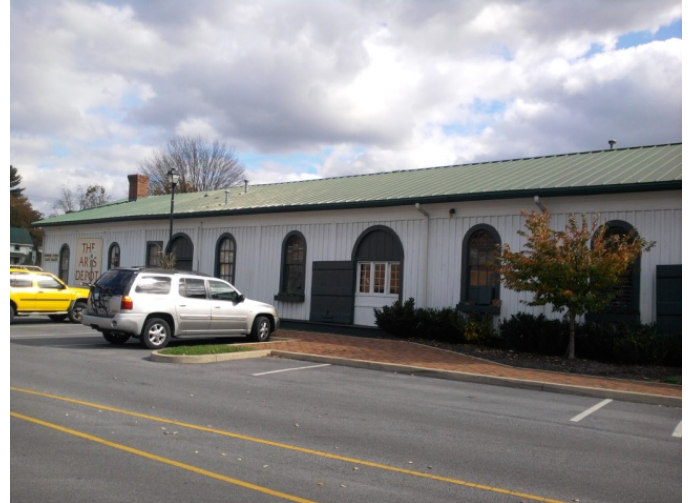
Freight House - Northwest Street Side
