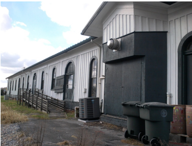
Freight House - South (trackside) Elevation
