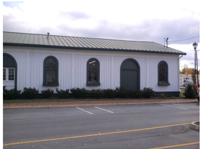
Freight House - Northwest Street Side
