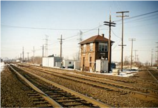
Signal box and tracks at Deval interlocking, Des Plaines, Illinois, in 1993
