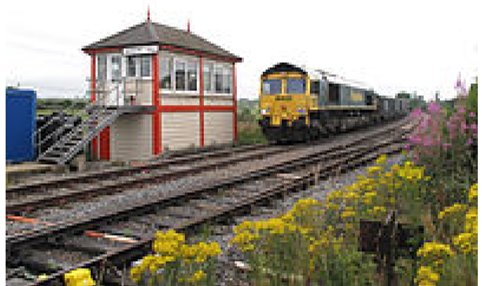
Bardon Hill box in England is a Midland Railway box dating from 1899, although the original mechanical lever frame has been replaced by electrical switches. Seen here in 2009.
