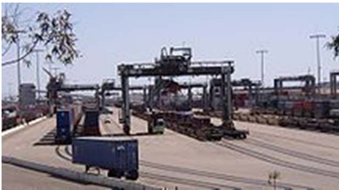
Intermodal ship-to-rail transfer of containerized cargos at the Port in Long Beach, California.
