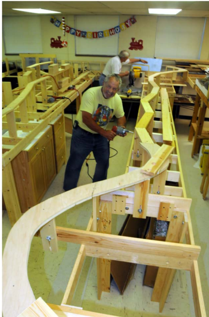
The new 1300-foot addition to the museum is rapidly being put to good use by volunteers, who are building a version of the narrow gauge East Tennessee & Western North Carolina (known affectionately as the Tweesie) from Johnson City to Cranberry, N.C.s ore banks. Four replicas of the railroad's engine as well as the special Hon3 track have been purchased; Museum President Dr. Fred Alsop looks up from his work finalizing support locations for the track, while member Dwayne Swank is custom-fitting the support system for the new track in the background.
