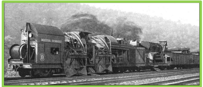
Track maintenance machine in action renewing ballast on the Pennsylvania Railroad.
