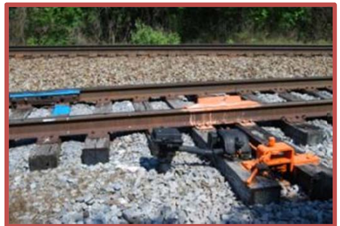
Modeler's Detail Derailer Installed on team track Jonesborough TN
