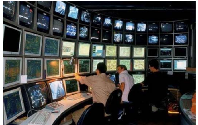
The whole system is controlled from a massive high-tech nerve centre.
