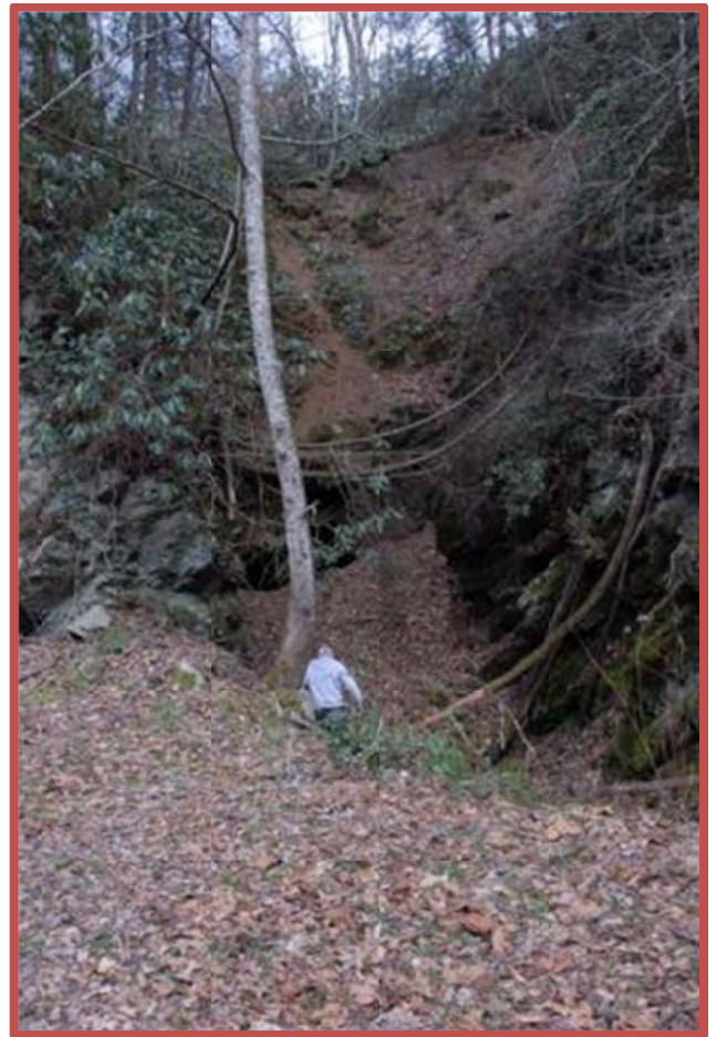
Photo 7: Rich Gallaher goes to explore the entrance of collapsed Sand Tunnel #5.
