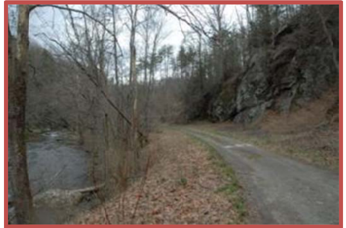
Photo 6: The Tweetsie ROW beside the Doe River north of Blevins between Blevins Steel Truss thru bridge and tunnel #5.
