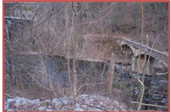
Photo 14: From the north side of the Doe River and from L to R: the new Hwy 19E/321 bridge, the ET&WNC north and south abutments for the covered deck bridge, and the old highway bridge connecting Elizabethton and Hampton, TN.
