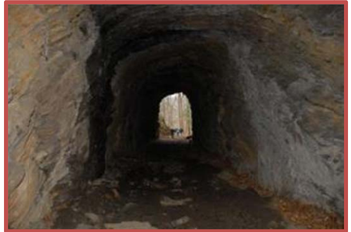
Photo 18: Inside short Tunnel #1 looking south.
