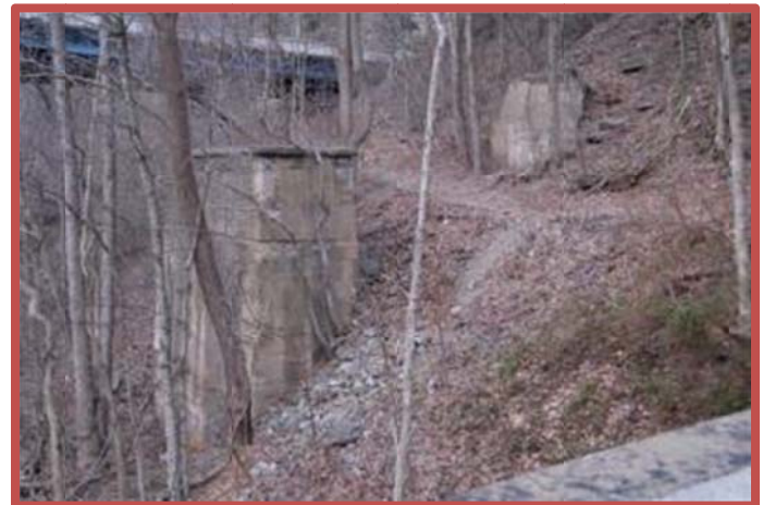
Photo 15. The poured concrete south abutments for the ET&WNC 3-span covered wooden deck bridge viewed from the old highway bridge.
