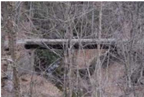
ET&WNC RR (former Linville River RR) Tank Trustle deck bridge near Vale, NC.
