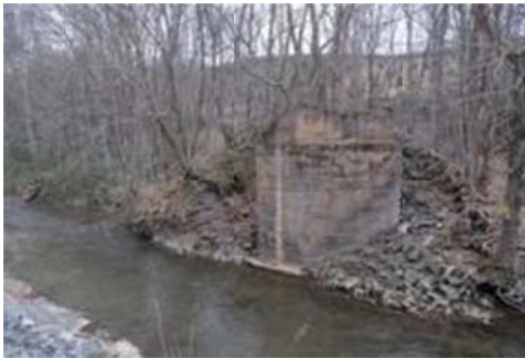
The concrete abutment for the ET&WNCRR (former Linville River RR) Tom Johnson bridge over the Toe River near Vale, NC
