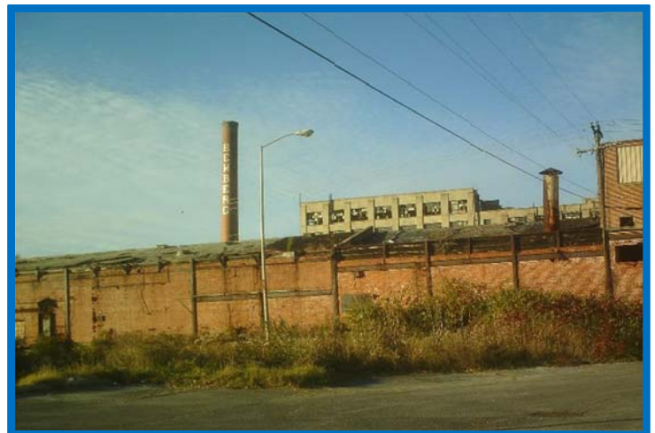
The Power Plant
