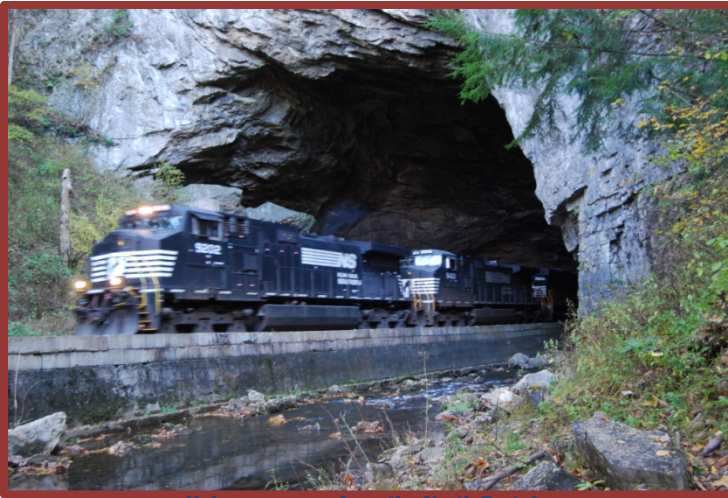
Helpers emerge from the North Portal
